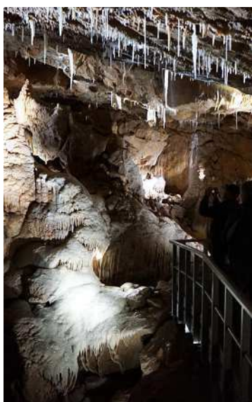
The FRP walkways show very little wear following 10 years of use. Track lights are well concealed within the handrails.
